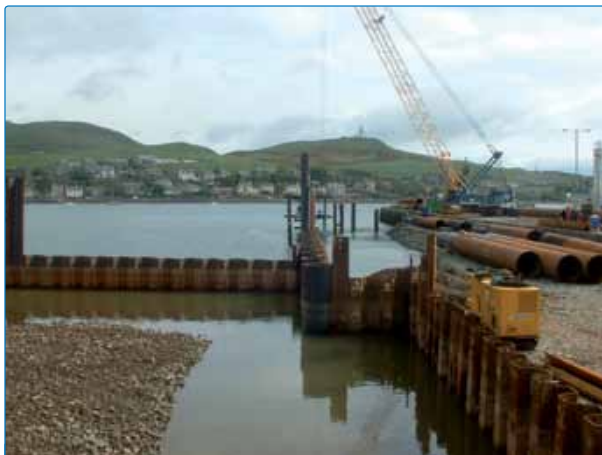
Figure 1. Typical steel combi-wall construction, Campbeltown Scotland.
